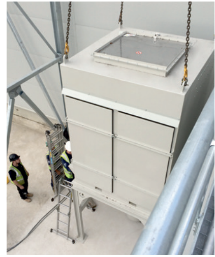
Crane lowering dust control unit into location
