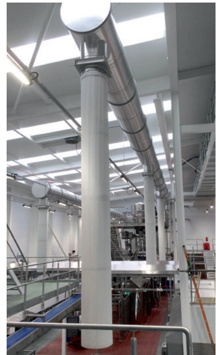
Aluminium ductwork with textile dropper assemblies
