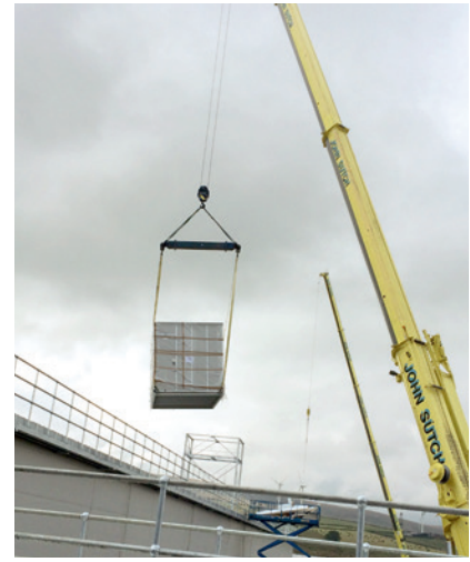
Crane lifting AHU section onto the platform
