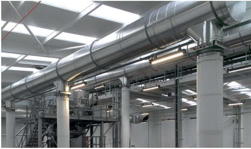
Aluminium and textile ductwork being installed on site
