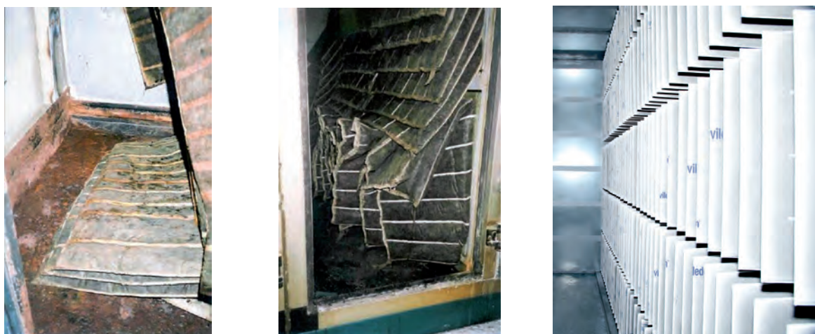
Figure 4-3: Wrongly installed pocket filters – horizontal (left and middle photos) and correctly installed pocket filters (right photo)
