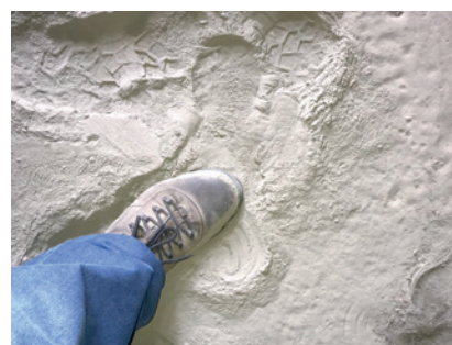
Initial situation: huge dust accumulation on filter house floor as a direct result of very high ambient dust concentrations
