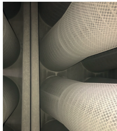
Installed Viledon® GTS cartridges after 20,000 hours in operation
