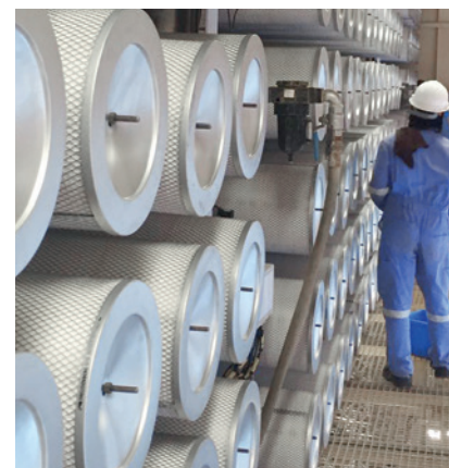
Installation of Viledon® GTS cartridges
