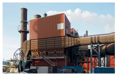
Bag filter house of Finnish steel manufacturer equipped with NEXX bags
